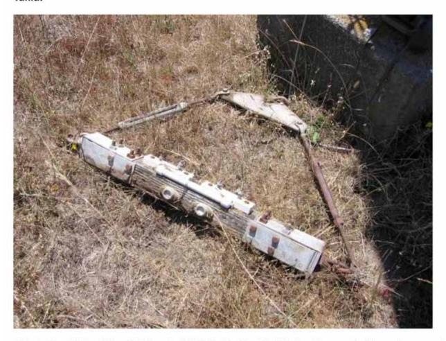
This is the bridle at the Tahiti end of R-209 - Made of 4x4 timber, it supported the antenna and provided a place for the terminating resistor, in the capped white tube, made with 4x4 timber! We will fabricate two new bridles from scratch to replace this one and the one still in the air at the feedline end of the antenna.
