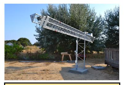
Top: the tiltable lower section of a Tasjian 52 fot tower during installation. Note that the top of the tower can be reached from a 10-foot step ladder.
