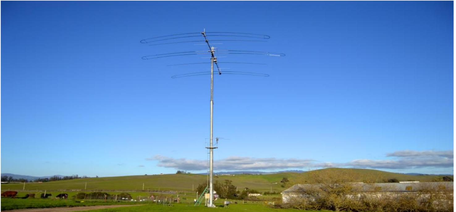
Pictured above is a SteppIR DB 42, the primary antenna at the N6IE remote site. The tower stands at 70 feet. The original tower was a 100-foot TriEx Sky Needle rotating tower that belonged to Frank Clement, W6KPC, the former owner of TriEx. Tashjian Towers did the rebuild. The llama is 3d from the left
