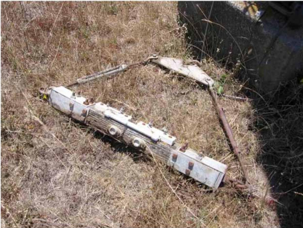
**This is the bridle at the Tahiti end of R-209** - Made of 4x4 timber, it supported the antenna and provided a place for the terminating resistor, in the capped white tube, made with 4x4 timber! We will fabricate two new bridles from scratch to replace this one and the one still in the air at the feedline end of the antenna.
