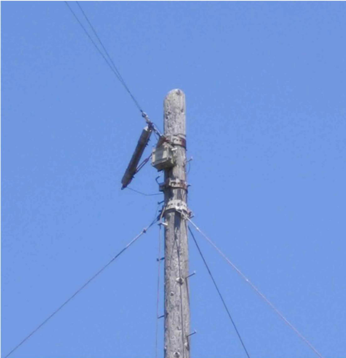
This is the bridle at the feed end of R209. It's still aloft - but barely. The curtain wires to the south are still connected. The ones to the north are gone (but recoverable on the ground). The antenna wires connect to a TMC balun, then to Heliax for connection with the receiver multicouplers.
