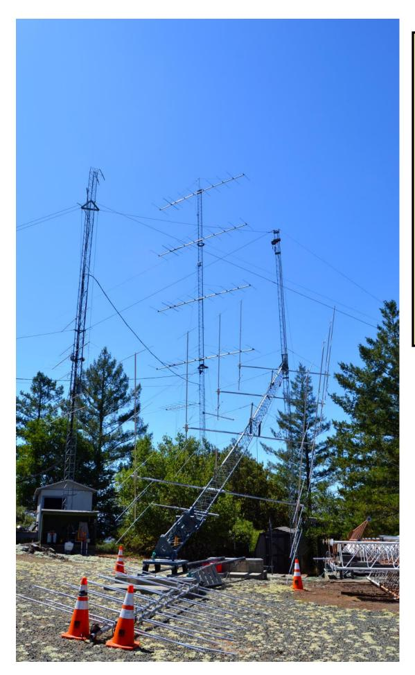
Part of the K6QXY antenna farm. In the foreground is the track on which the base of the antenna moves to change elevation. All EME QSOs require settings for azimuth and elevation.
